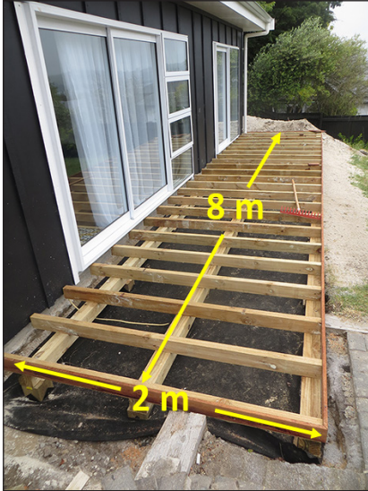
Deck measuring 8 metres \times 2 metres
