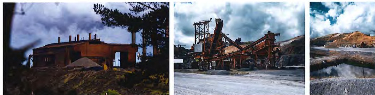
The Scale of the Glenbrook Steel Mill
